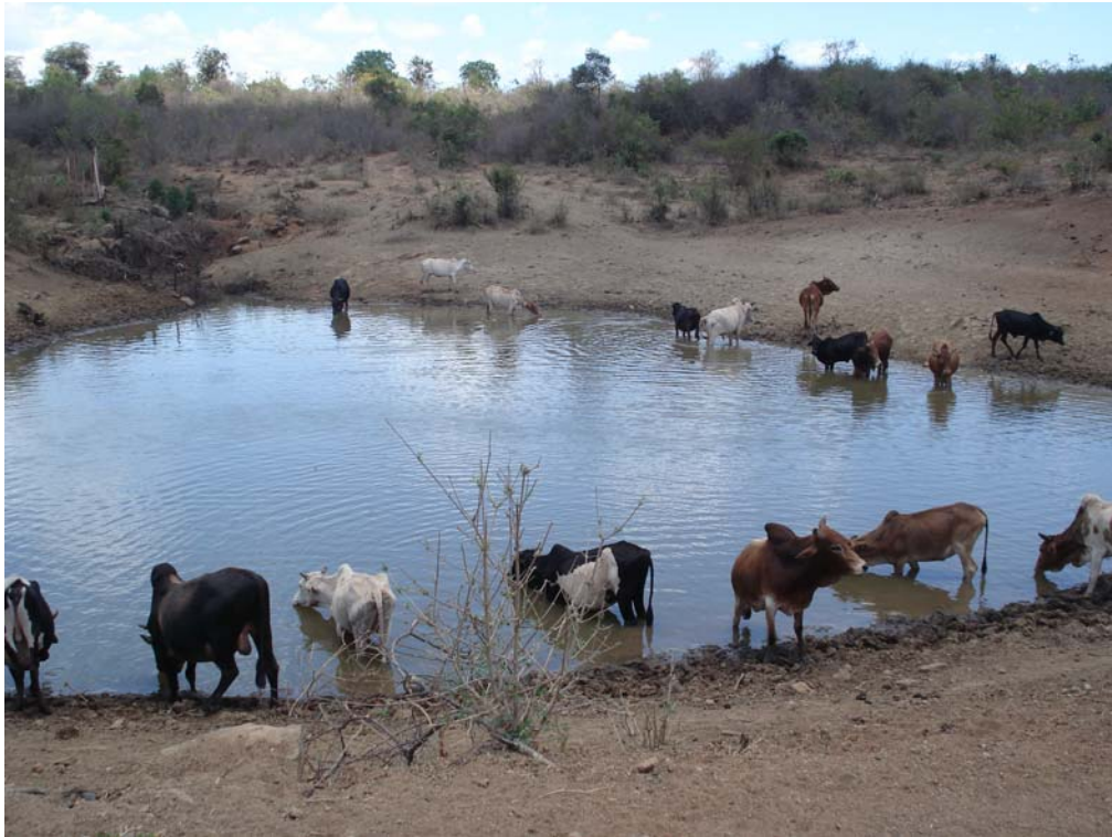
Plate 15: Unprotected earth dam with livestock watering inside
