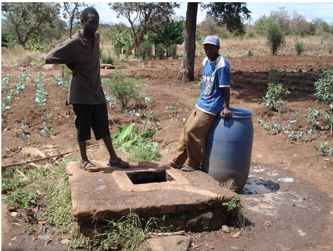
Plate 8: Shallow well that uses bucket and rope abstraction method
