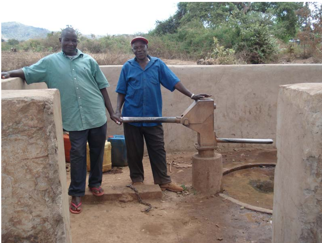
Plate 12: Concrete wall to protect the borehole
