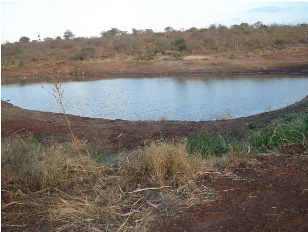
Plate 13: Fenced earth dam to keep livestock away
