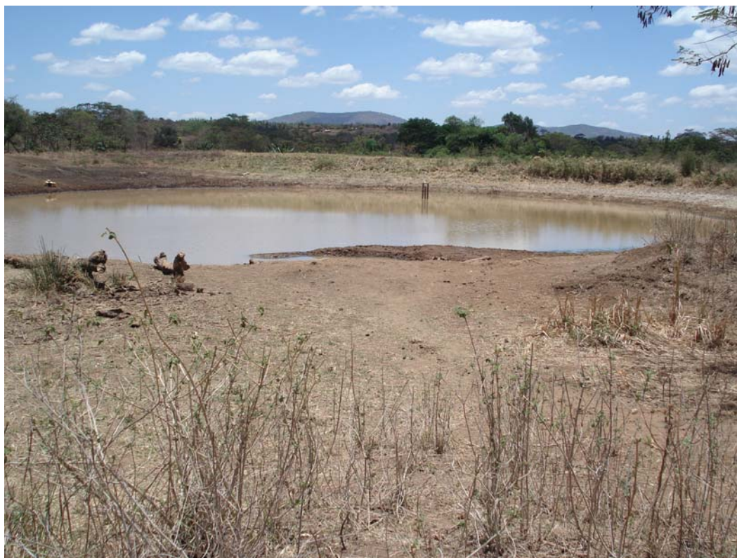
Plate 4: An Earth dam
