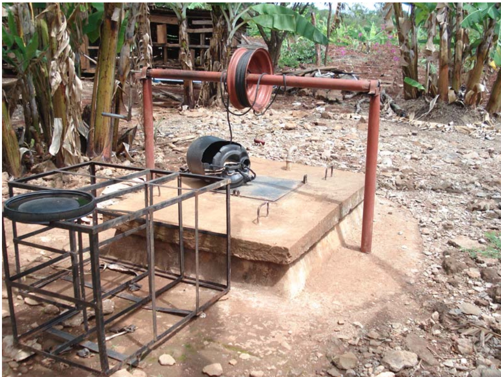
Plate 16: Concrete covered well to keep water clean
