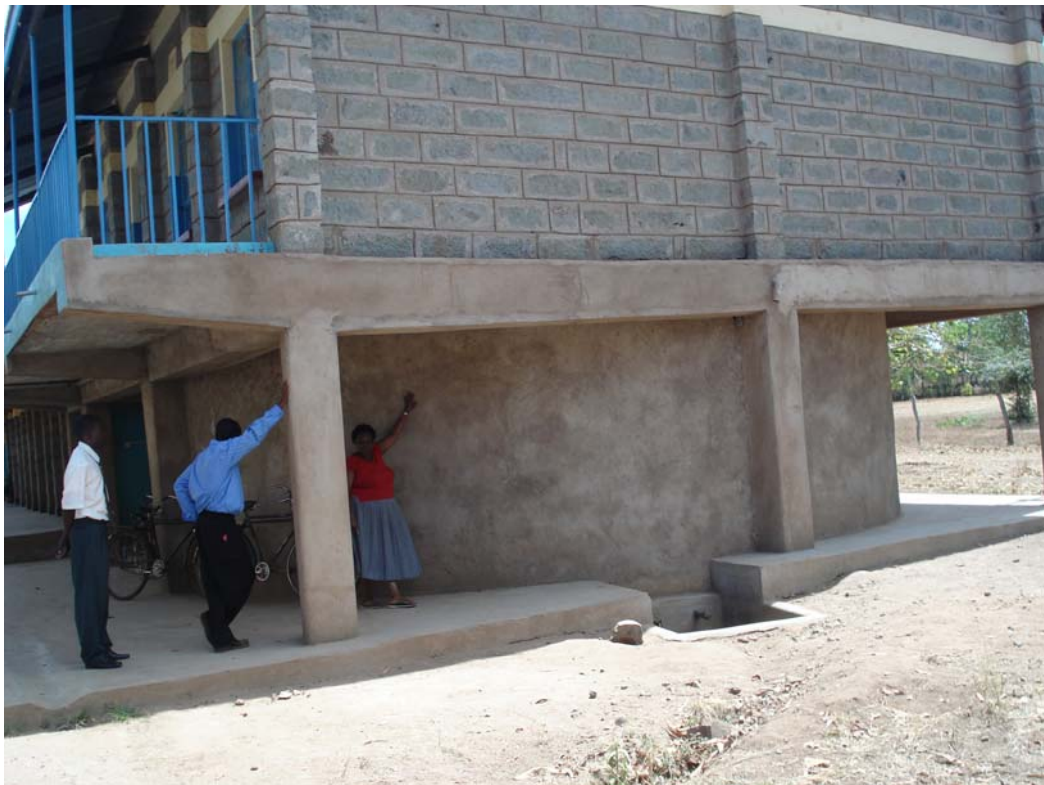
Plate 3: Roof water harvesting to a storage tank beneath the building
